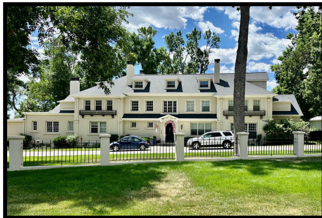
17 Broadmoor Ave., Built 1905 Broadmoor Neighborhood
