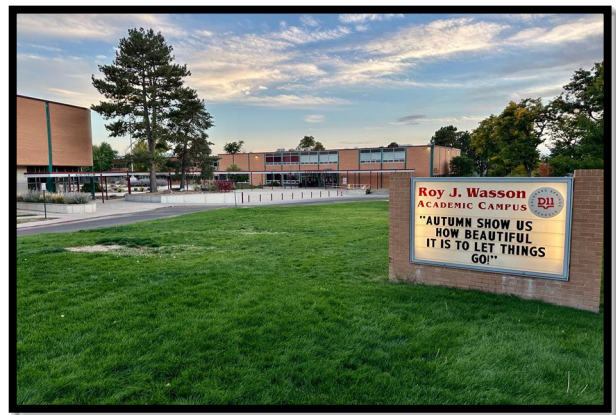
Wasson High School, Built 1959 2115 Afton Way
