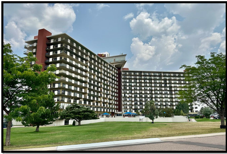
Satellite Hotel and Condominiums, Built 1968-1974 411 Lakewood Circle
