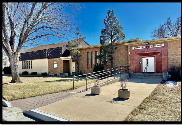
Temple Shalom, Built 1951 1523 E. Monument St.
