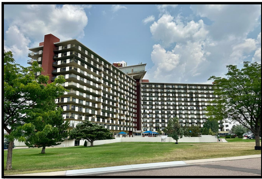
Satellite Hotel and Condominiums, Built 1968-1974 411 Lakewood Circle
