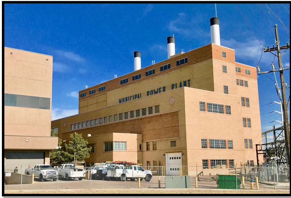
Municipal Power Plant, North Nevada Avenue, Built 1953
