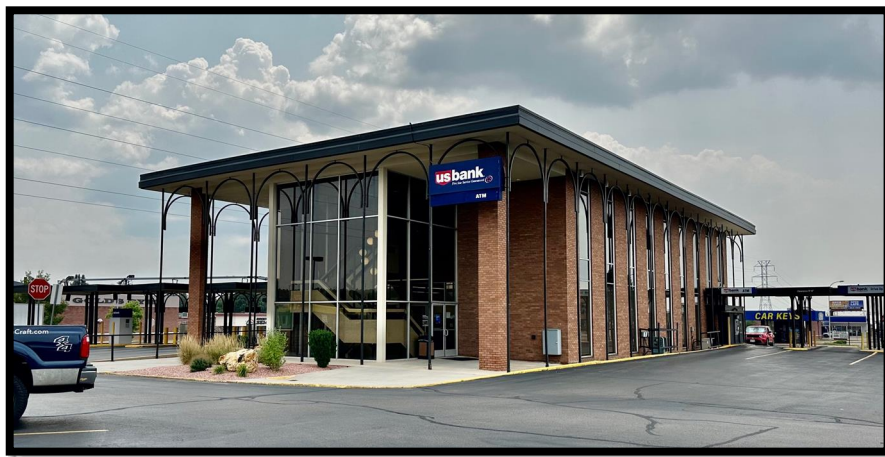
US Bank, 1415 N. Academy Blvd., Built 1965
