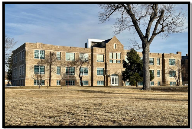
Gottlieb School Building, Built 1952
