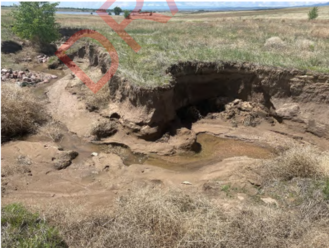
Figure 7 (Station 4+50): Bank failure within reach (looking downstream)
