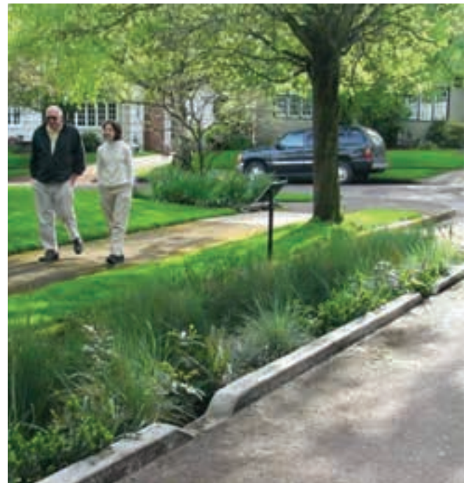
Low Impact Development (LID) infrastructure adds beauty, storm water mitigation and water quality improvements to neighborhood streets as shown in Portland, Oregon.
