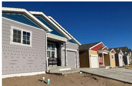
New Habitat for Humanity home under construction Photo credit: KRDO Grocery Services
