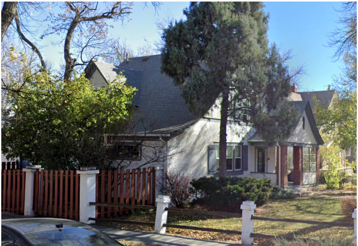
Existing House View form the Corner of Nevada & Jefferson
