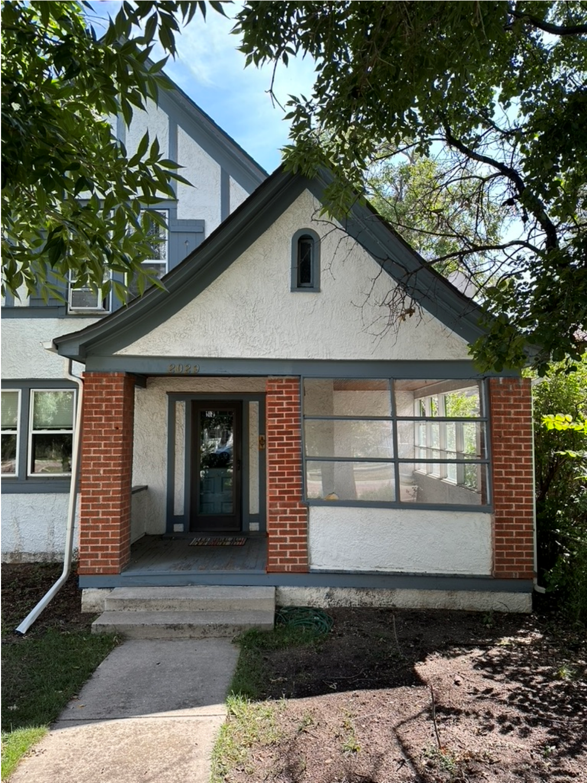
Existing house and porch
