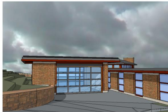
NORTHWEST ENTRY DRIVE VIEW
