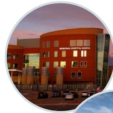
Memorial Hospital North
