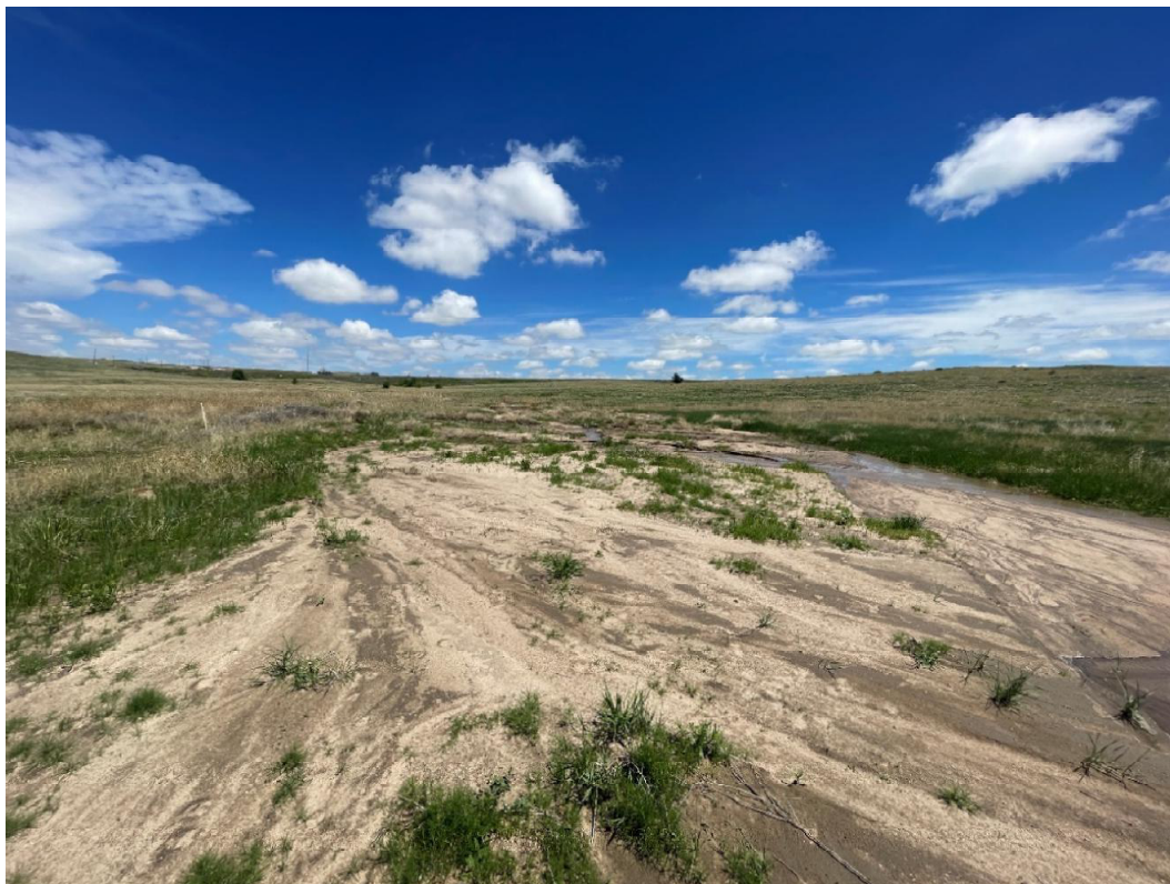
Figure 11(Station 14+00): Wide alluvial wash (looking upstream)
