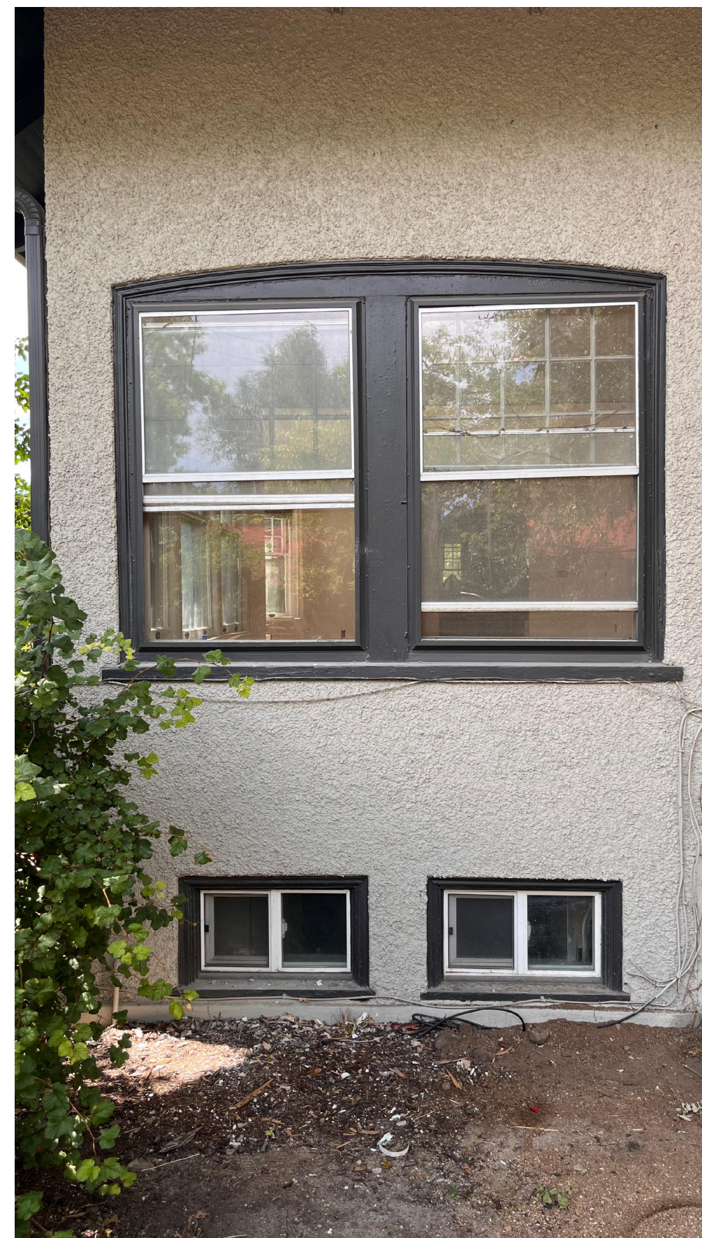
3 A-2 EXISTING EAST WINDOWS
