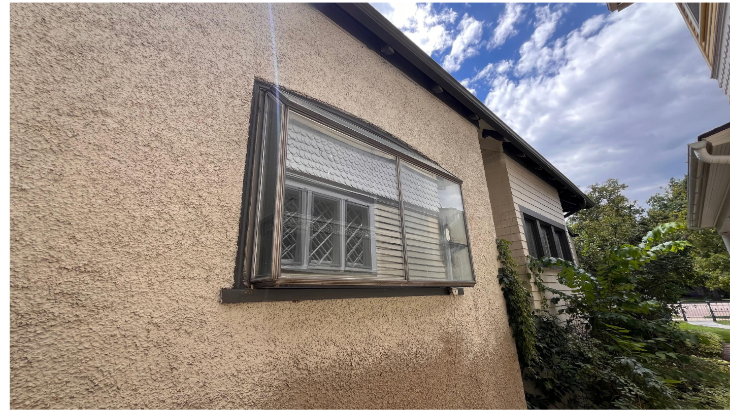
2 A-2 EXISTING NORTH WINDOW
