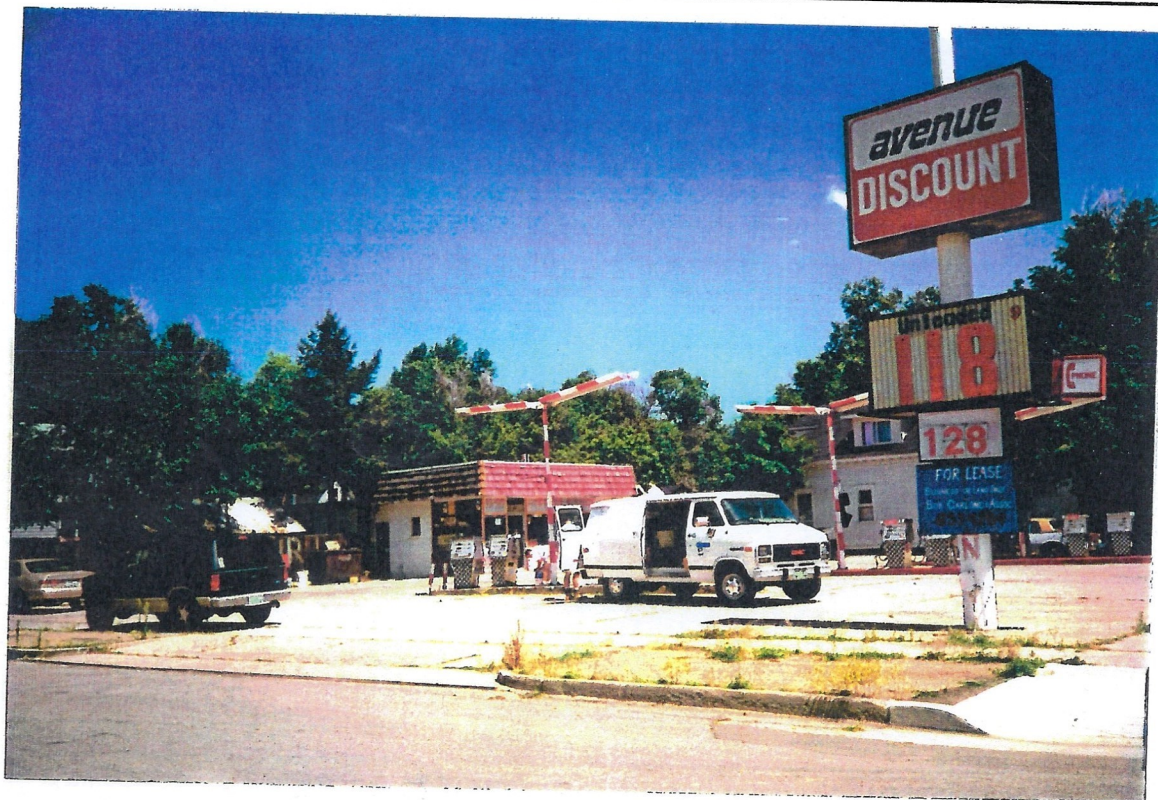
Northeastern view of Avenue Discount Gas Station from 9th Street
