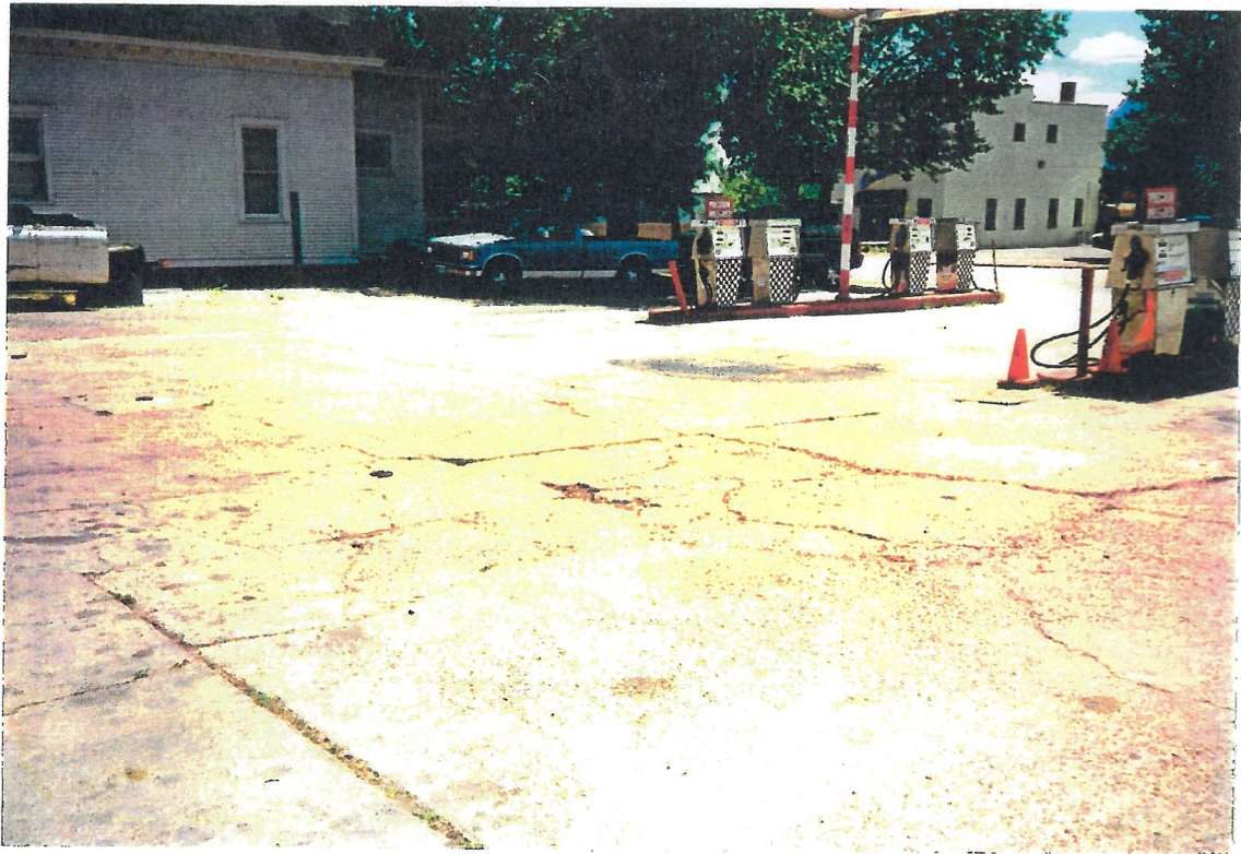
View of parking area and location of the three 8,000 USTs, (left to center of photo)
