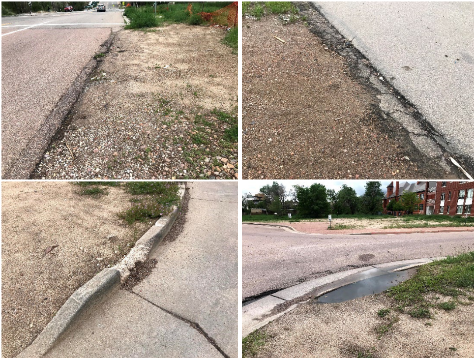
Figure 8. Deteriorated Curbs
