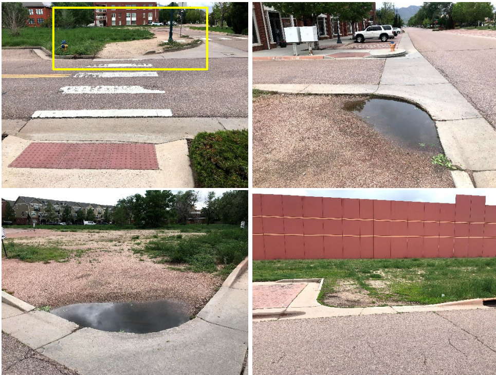
Figure 3. Lack of Sidewalks
