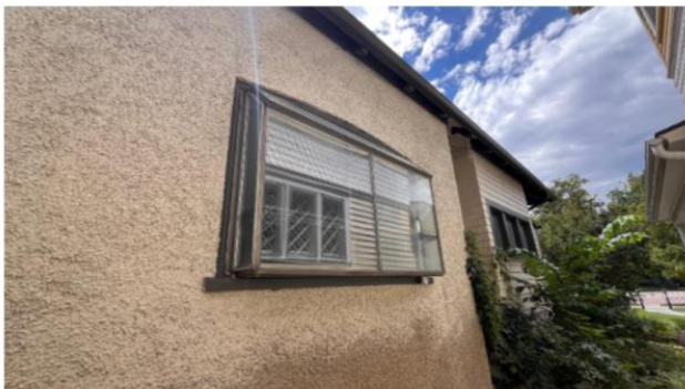
2 A-2 EXISTING NORTH WINDOW
