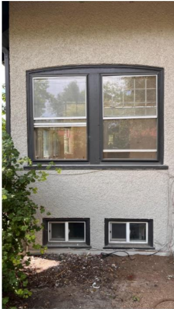
3 EXISTING EAST WINDOWS A-2
