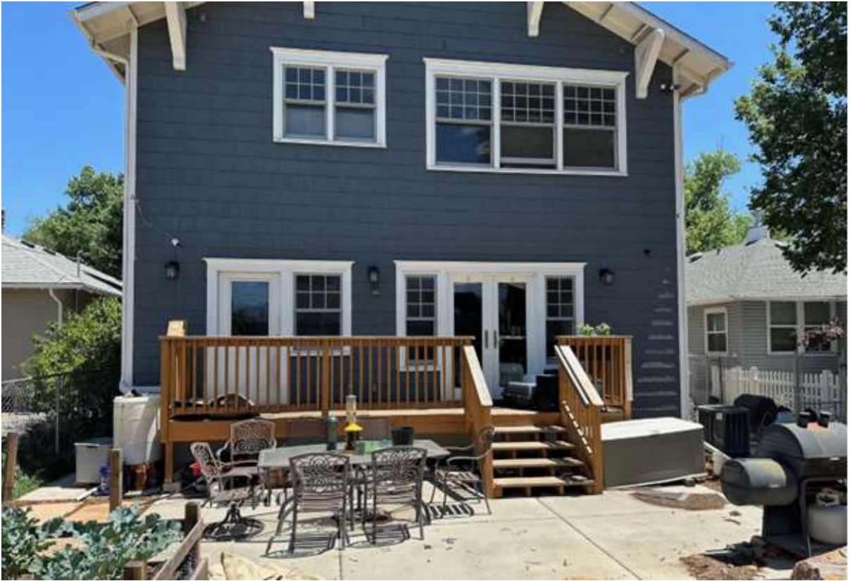
Existing rear landing
