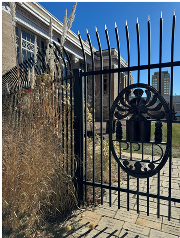
Existing fencing at Penrose Library
