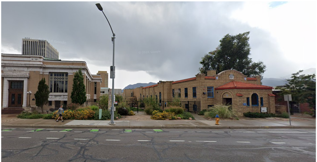
Existing fencing at Penrose Library Along W. Kiowa St
