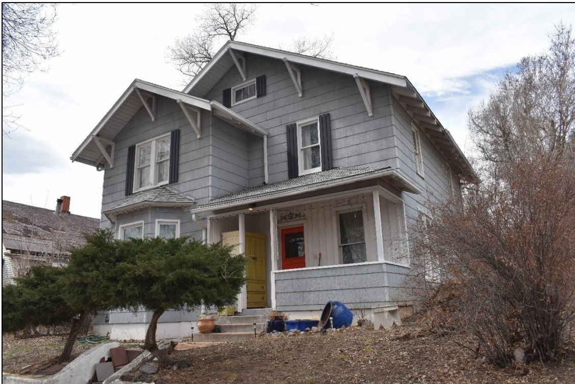
10 of 11. The front and part of the north wall from the sidewalk, showing the porch detail. View west-southwest.
