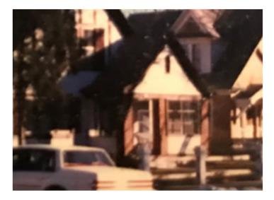
A key characteristic of historic homes in the Old North End are their porches, mostly always raised. The existing porch is raised approximately 10" to match the threshold of the front door. The primary historic elements are the roof shape, supports, railing and baluster detail. Glazing and a solid pony-like wall are not elements of front porches. The Interpretive Guide for Old North
