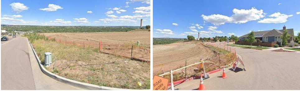
Figure 4. Poor Provision of Street Improvements for Pedestrians
