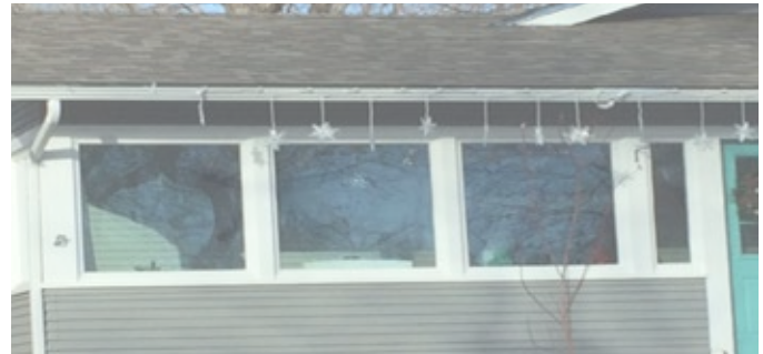
AVOID enclosure of open porches with unbroken walls and large windows of incorrect proportions.
