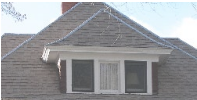
RECOMMEND window replacement that fits within the existing dormer element.
