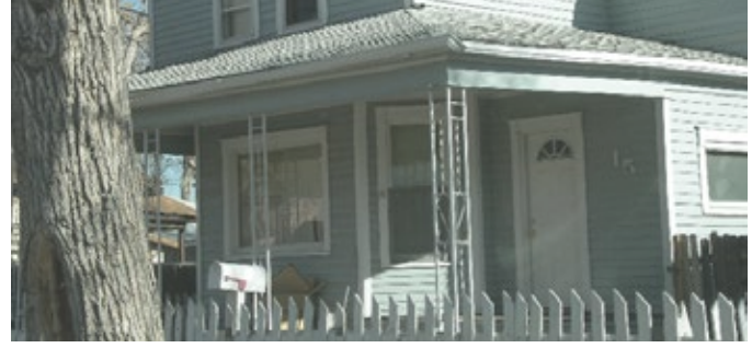
AVOID the use of thin tubular metal support columns on pre-war styles of homes unless historic evidence shows their appropriateness. They were commonly used for a time on post-war homes.
