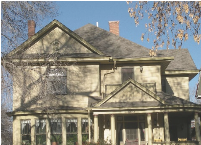
Edwardian style home with multiple gable elements and a primary hip roof.
