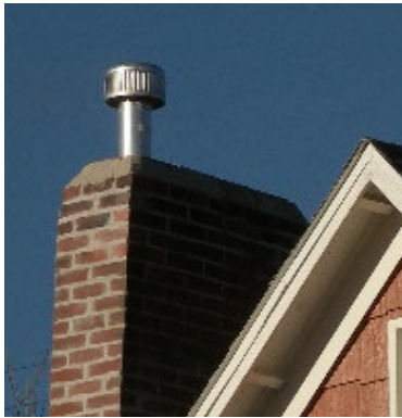
Brick masonry chimney with flue liner and modern termination cap flue.
