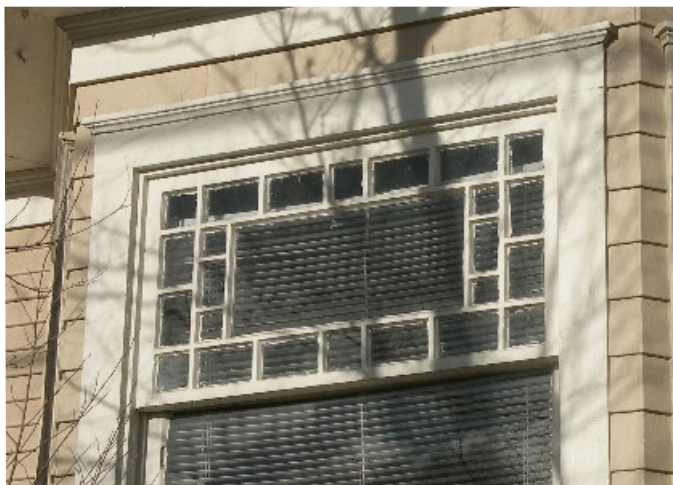
Ornate preserved wood transom window with multiple small panes divided with wood muntins.
