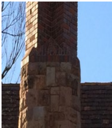
Original stone masonry chimney.
