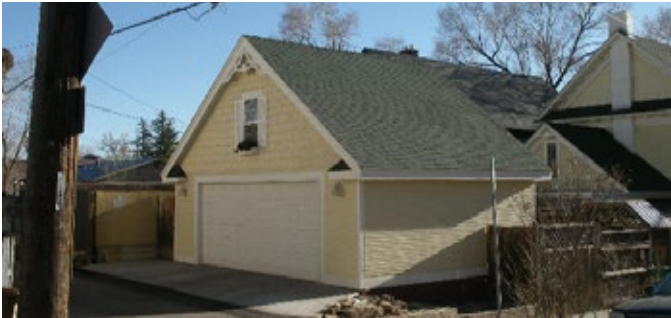
RECOMMEND new structures be designed to replicate forms of primary structures including roof pitch.
