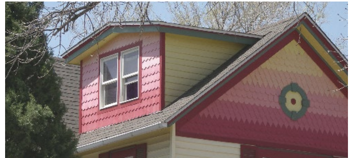
Dormer addition roof slope does not match primary roof slope but is subordinate to main ridgeline.
