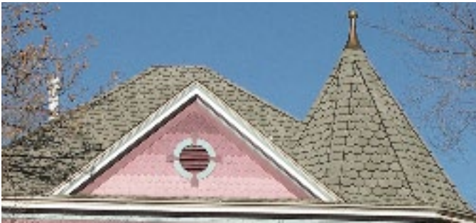
RECOMMEND the use of decorative shingles for accents and design variety where there is historic evidence they were used on this building or where reference books show historic usage in a similar application.
