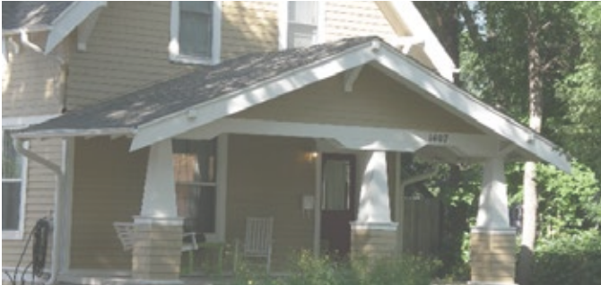
RECOMMEND new supports that are appropriate to the style and era of the house. This Craftsman style home received new tapered columns on shingled bases to match the style and siding.
