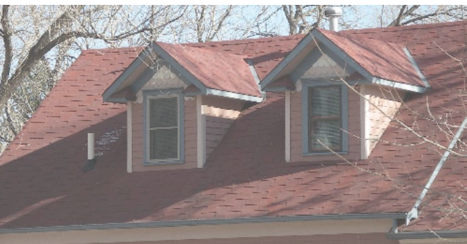
RECOMMEND that new dormer elements replicate historic forms and are subordinate to main roof.
