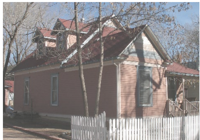
Two story addition appended to rear of existing one-story structure. New roofline is higher than existing but slope and dormer details match the original. New materials were selected to match the historic original materials.
