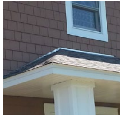
Flashing behind siding
