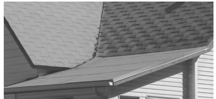
AVOID the use of roll roofing when the roof slope is of adequate slope to use shingles that match the main roof.
