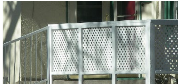
AVOID the use of lattice for balusters. Lattice is appropriate for crawlspace enclosures and trellises.
