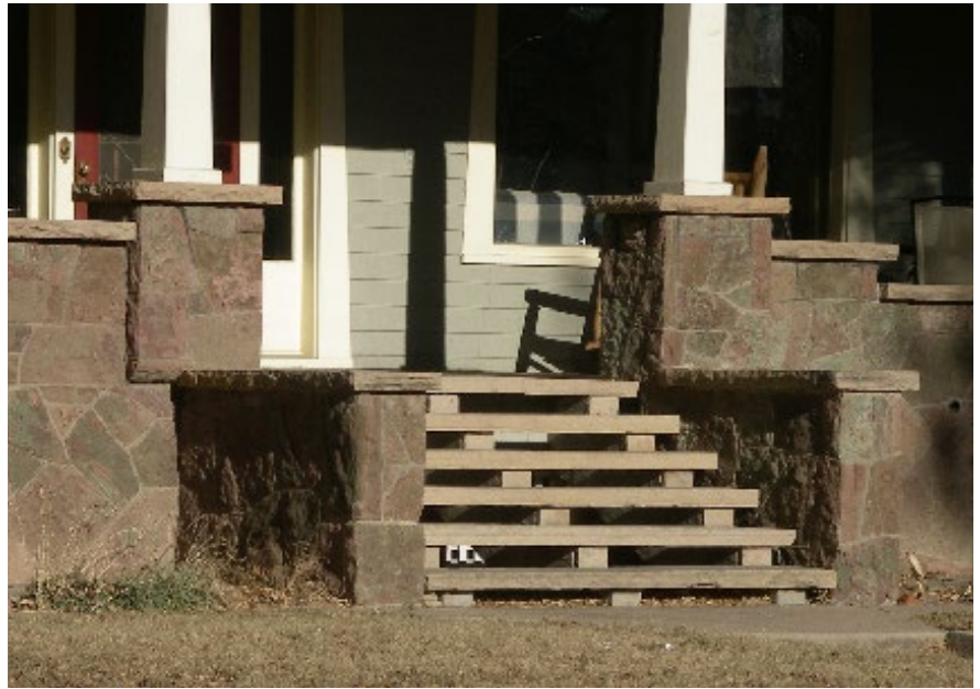
Manitou greenstone masonry porch wall with slab stone stairway.
