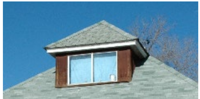
AVOID window replacement that does not replicate the historic window type or trim and siding type.
