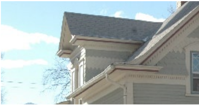
RECOMMEND retaining original roof dormers in their historic condition.
