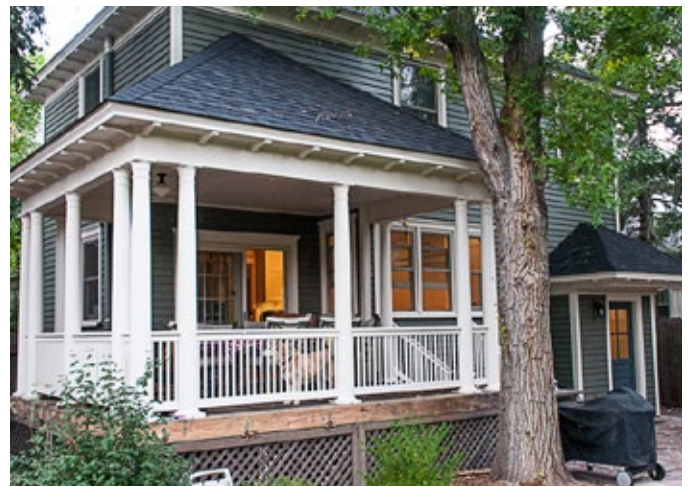
Example of the back porch of house pictured below left. Porch balustrade and column features provide recommended unity with front porch of house.
