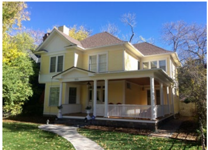
After: Completed renovations exhibiting new porch, landscaping and exterior paint.
