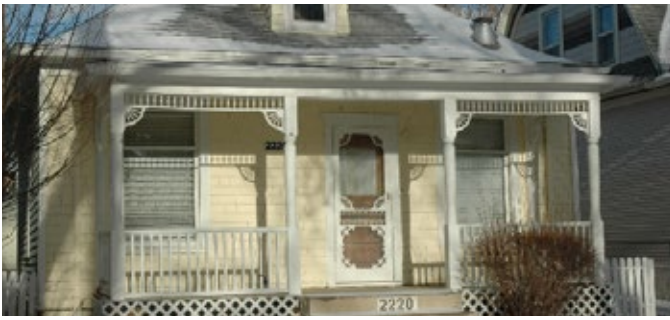
RECOMMEND preserving and rehabilitating existing historic porches and detailing.
