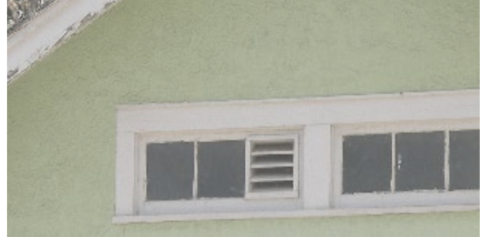
AVOID installing vents that do not fit with existing openings or that remove existing trim or siding.
