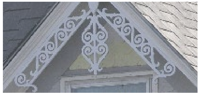
AVOID installing excessive ornament unless there is historic evidence that it was originally present.
