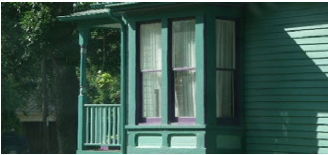
RECOMMEND preserving and repairing existing historic windows.
