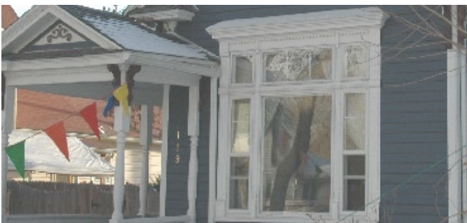
RECOMMEND storm windows using wood sash or prefinished aluminum to match profile.
