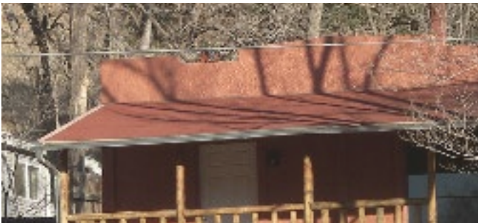
RECOMMEND matching roll or color membrane roofing on low slopes only where shingles cannot be used.
