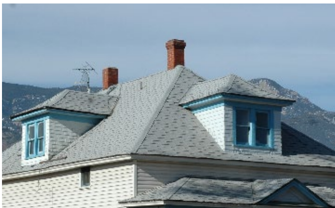
Classic Cottage with hip roof dormers to match the primary hip roof.
