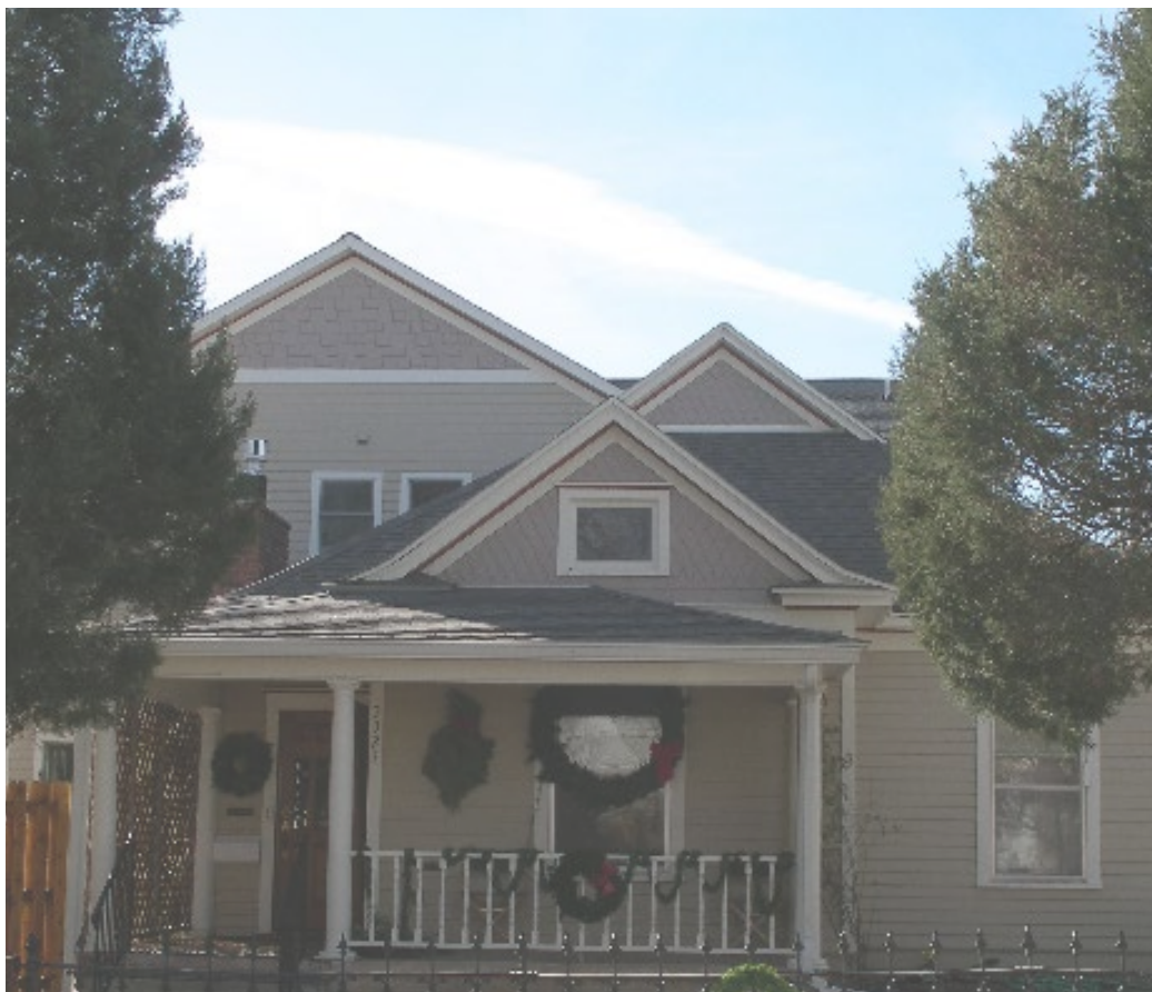
Large two-story addition constructed to the rear of existing historic house. Design retains front portion of existing structure and utilizes similar roof slopes and detailing for new portions on the left side of the house.
