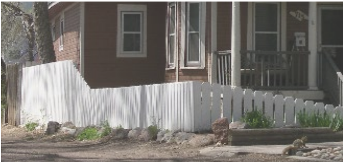
RECOMMEND stepping high side and rear yards fences down in height at front yard areas.
