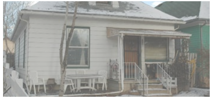
AVOID demolishing and replacing historic porches when elements remain to allow reconstruction.
