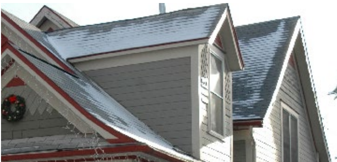
RECOMMEND using restraint when adding new ornamental or accent siding areas unless existing detailing on the building is being followed.
