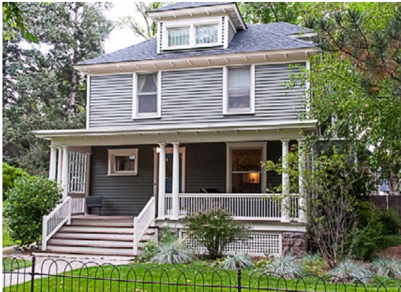
Example of restored porch, railings, and columns to historical accuracy.
