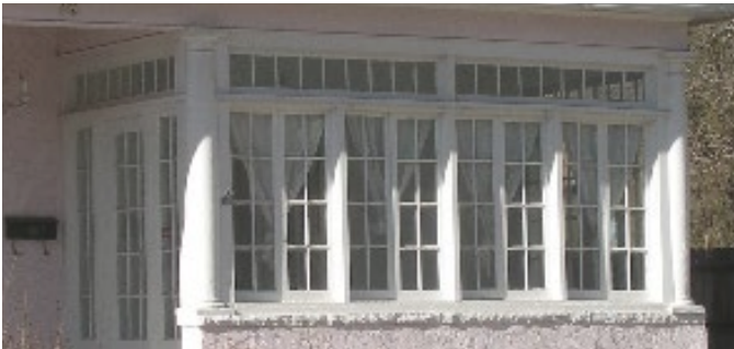
RECOMMEND that partial porch enclosure panels utilize glass instead of solid surfaces.
