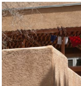
New colored stucco exterior wall finish.
