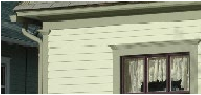
RECOMMEND retaining original trim widths and detailing at building corners.
