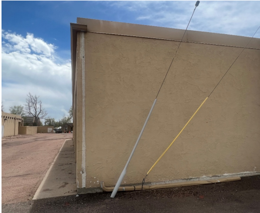
Figure 3. Deteriorated Gutters/Downspouts
