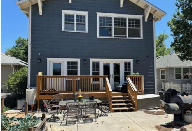
Existing rear landing
