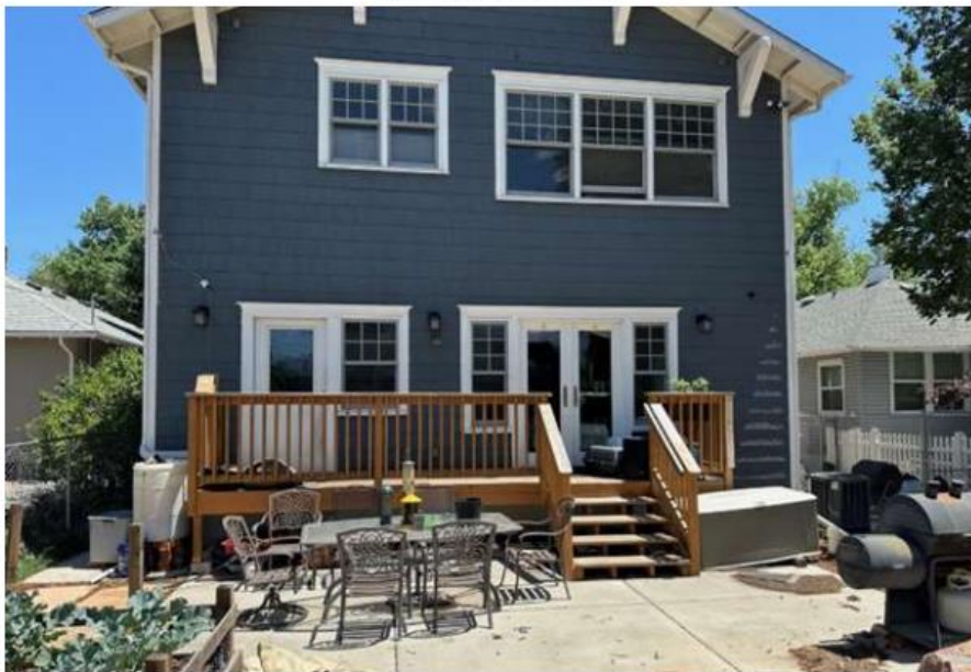
Existing rear landing
