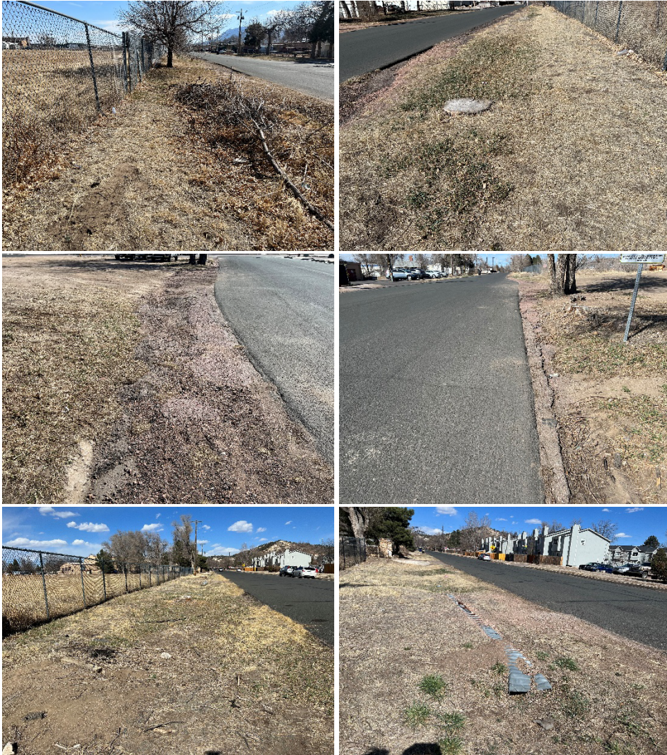
Figure 9. Lack of Curb, Gutter/Drainage, and Sidewalks
