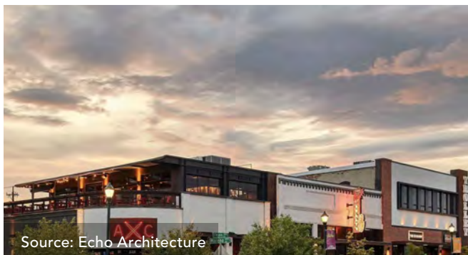
The Trolley Block transformed former trolley warehouses into a vibrant mixed-use district.
