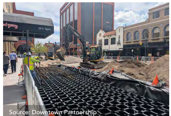
Soil cell installation along Tejon Street
