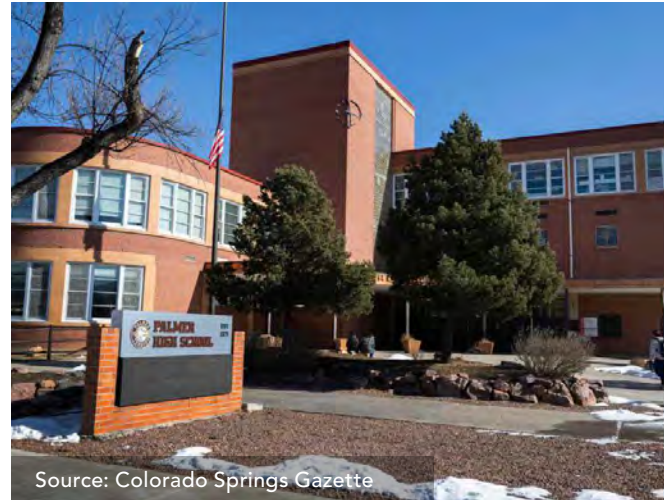
Palmer High School renovations have begun, marking a new era for collaboration and opportunity for students and the broader Downtown area.
