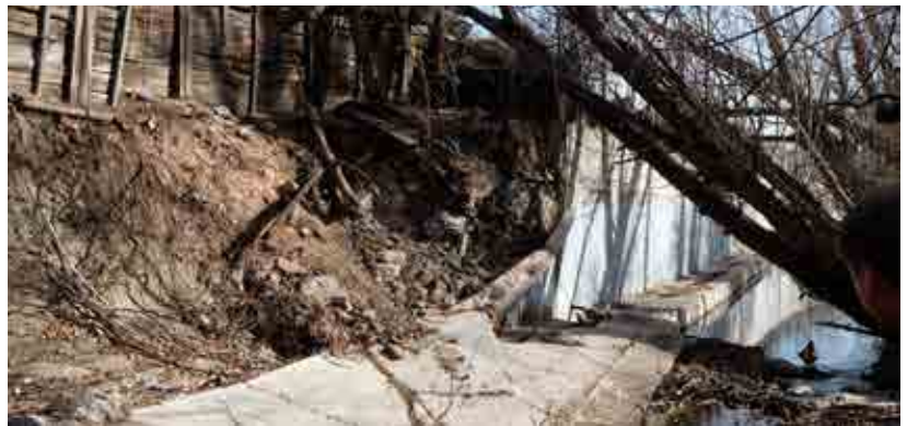
Failing retaining wall along Corridor pathway
