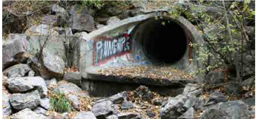
Erosion below a tributary drainage outlet along Shooks Run
