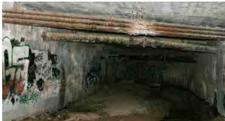
Utilities passing through structure at Cache la Poudre Street
