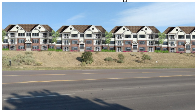
AFTER: Northeast corner along N. 30 th Street.
