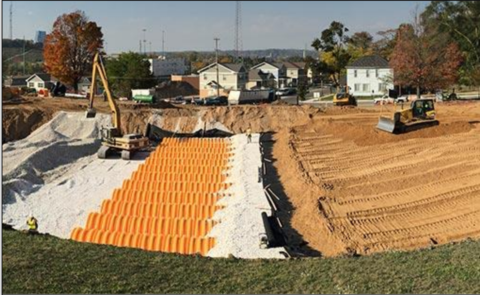
Photograph of subsurface StormTech stormwater chambers
