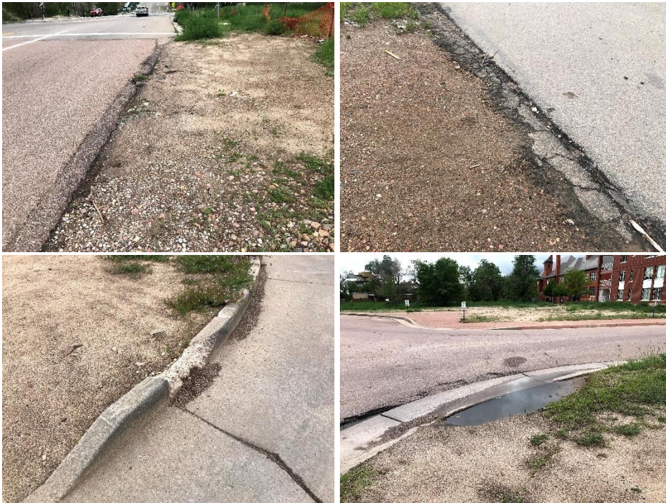
Figure 8. Deteriorated Curbs
