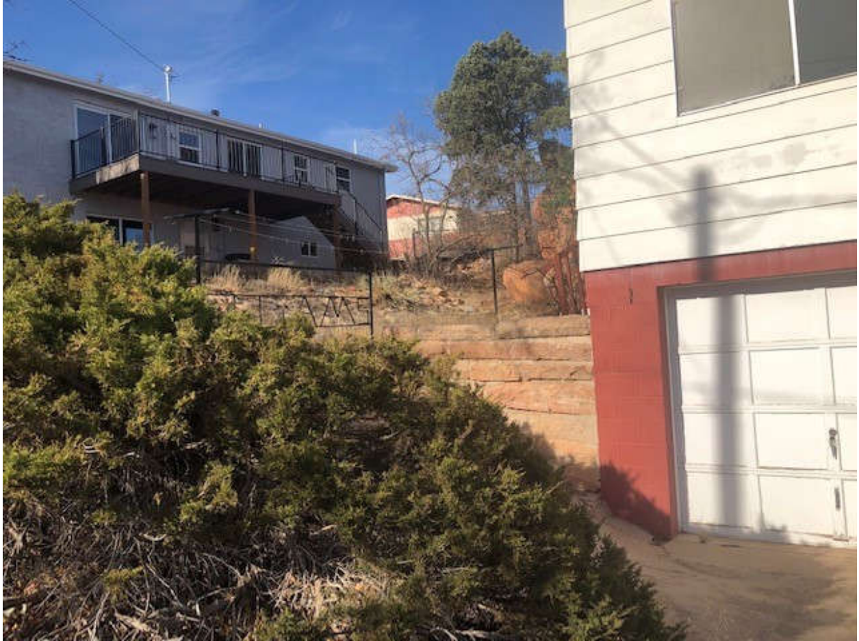
Retaining wall, west of detached garage to remain
