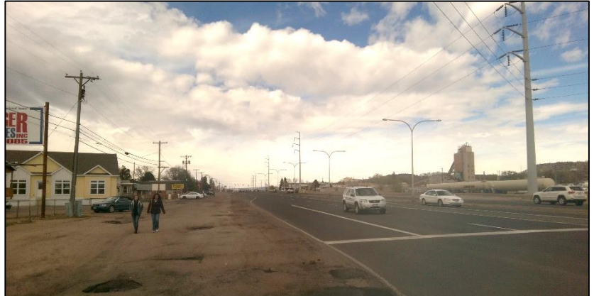
The lack of curb, gutter, sidewalk and access control creates conflicts and safety issues
