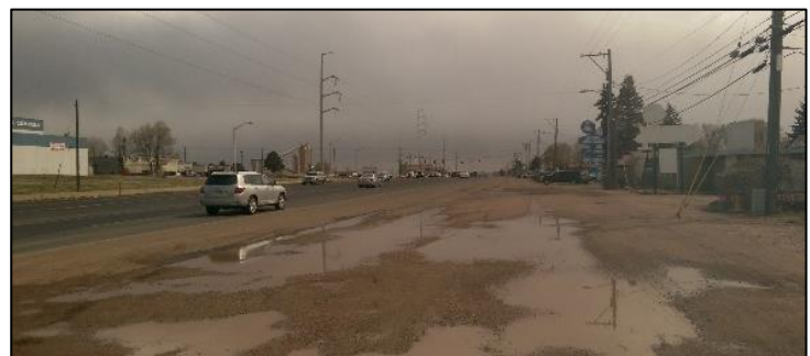
Evidence of inadequate stormwater infrastructure in the corridor
