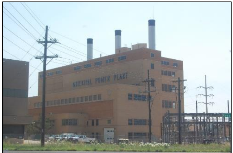
Birdsall Power Plant
