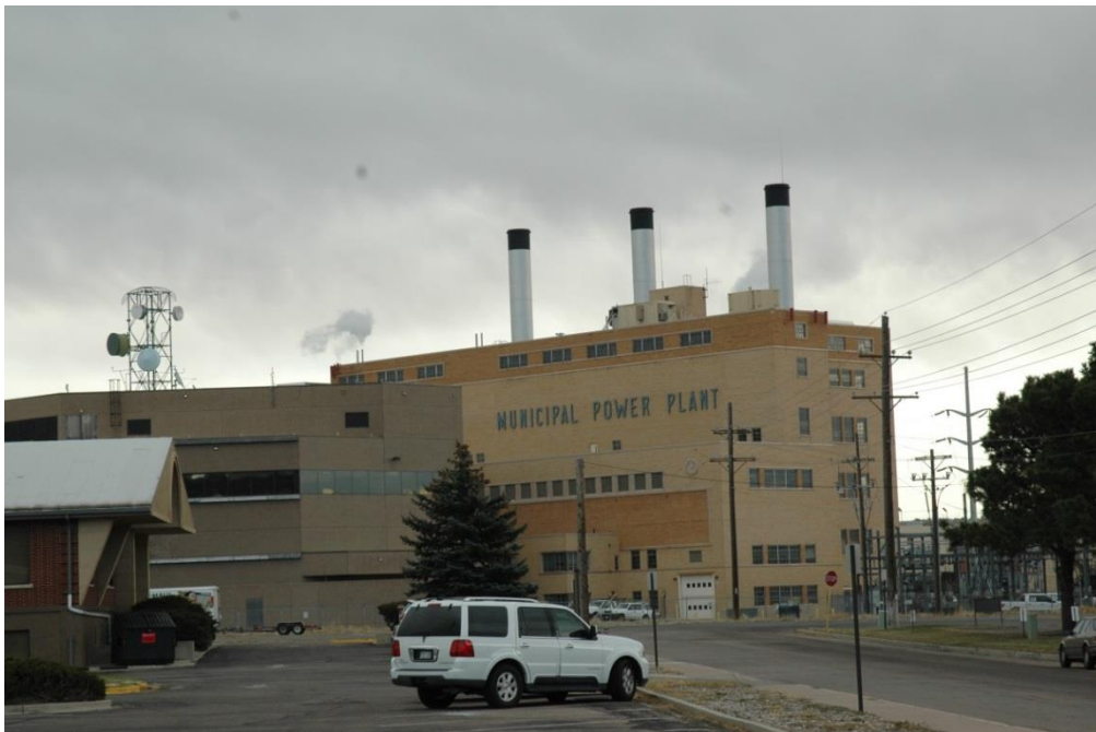
Photo 5- Birdsall Power Plant
