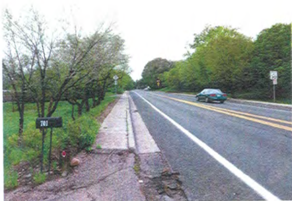
Looking South Along Cresta Road
