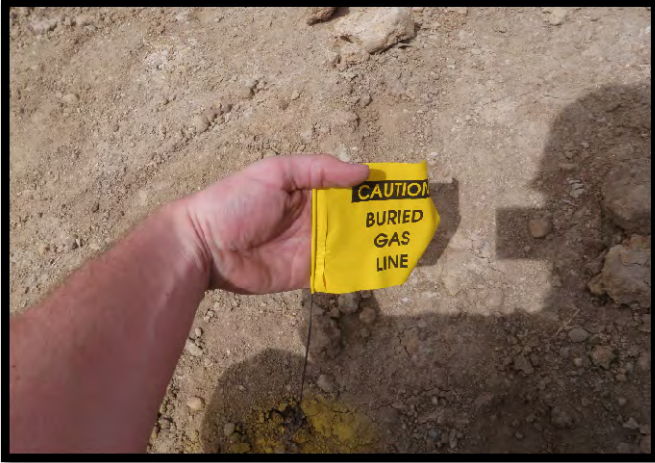
Gas line evidence
