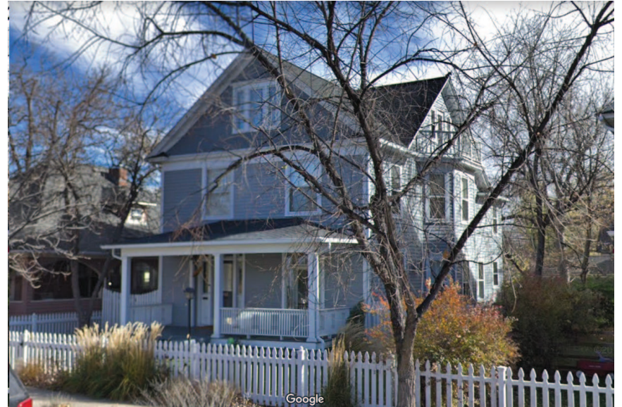
Closer view of front of home from the south
