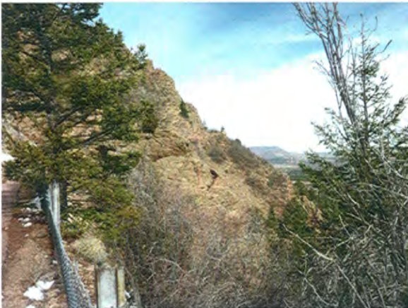
Looking North Across a Portion of the Larger Parcel From Cheyenne Hwy
