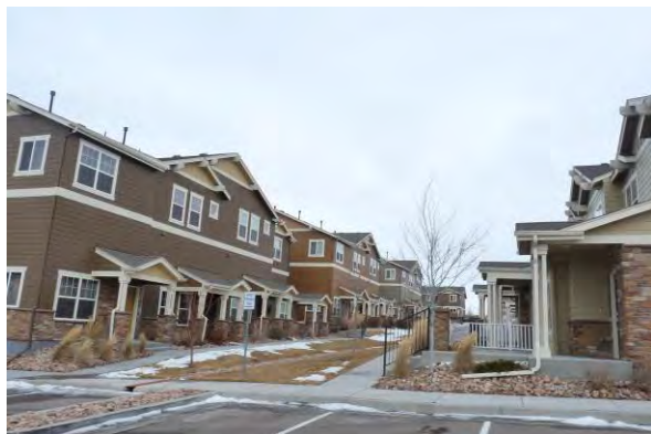
Typical Dublin Terrace Townhomes
