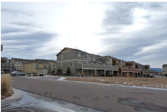
Typical Dublin Terrace Townhomes
