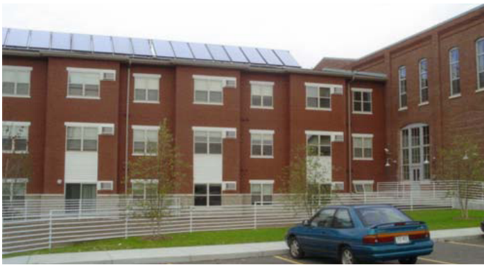
New rear addition with rooftop solar panels.
