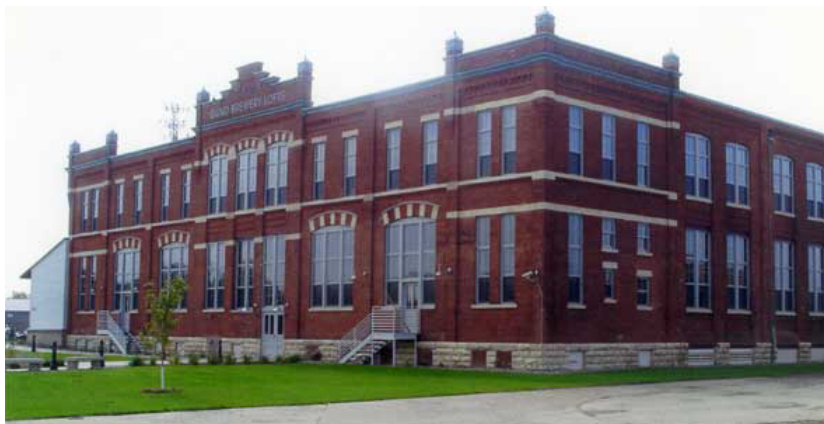
Primary view of the brewery after rehabilitation.
