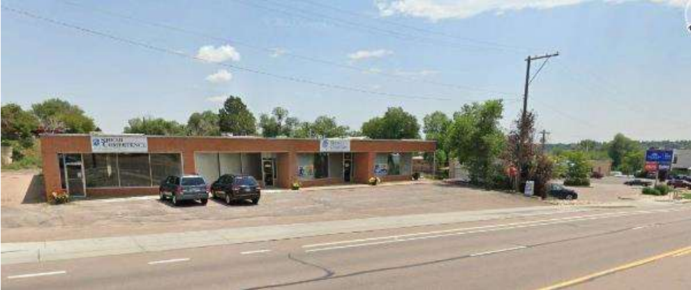
Strip Mall – 1407 8 th Street
