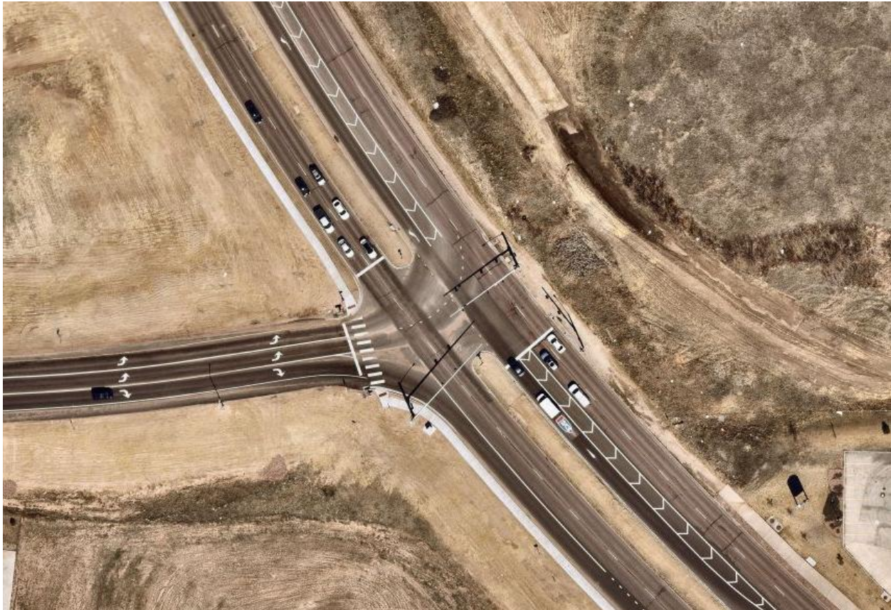
Powers Boulevard Off-Ramp and Voyager Parkway (#6)
