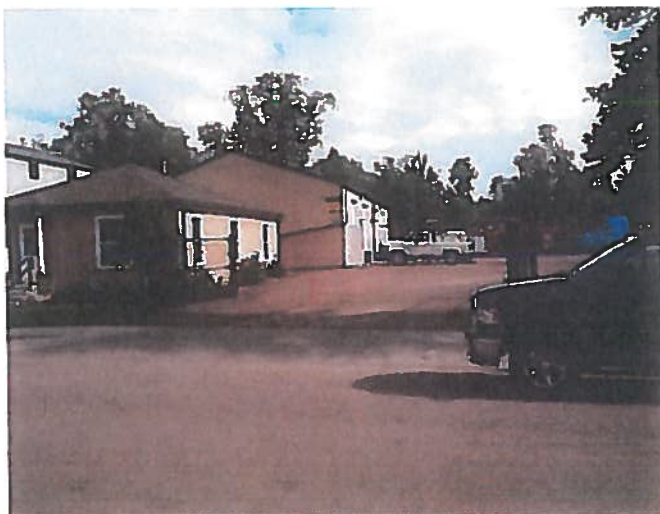
Colorado College's current warehouse
