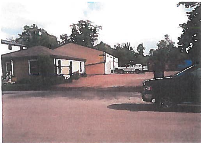
Colorado College's current warehouse
