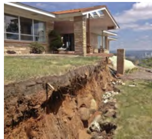
Photo: Constellation drive landslide, Colorado springs, August 2015. Source: T.C. Wait, Colorado Geological Society
