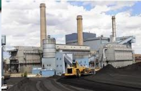
Martin Drake Power Plant #5 – (46 MW) #6 – ( 77 MW) #7 – (131 MW) Site total Energy (254 Mw)
