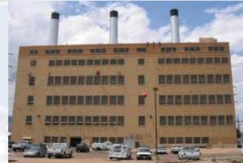
Birdsall Power Plant Steam Cycle Natural Gas Plant (55 MW)
