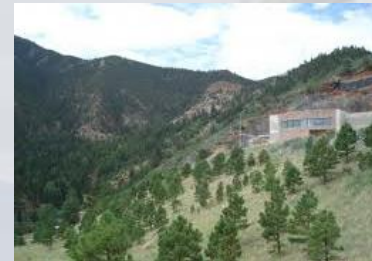
Total CSU Hydro Electric plants (35 MW)
