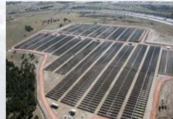
Contracted Solar Facilities Air Force Academy Solar Array (5 MW) Solar Gardens (1MW)
