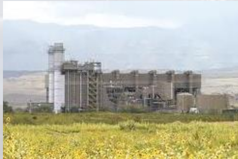
Front Range Power Plant – Combined cycle natural gas plant (460 MW)
