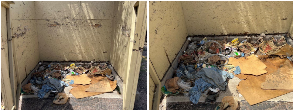
Figure 8. Evidence of Vagrants
