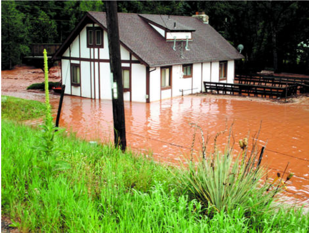
Figure 1. Fountain Creek inundates homes in Green Mountain Falls.
