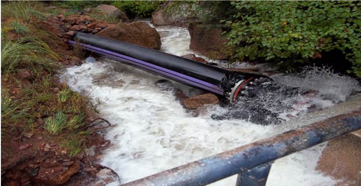
Figure 7. Colorado Springs Utilities raw water intake near Manitou Springs damaged by floodwaters.
