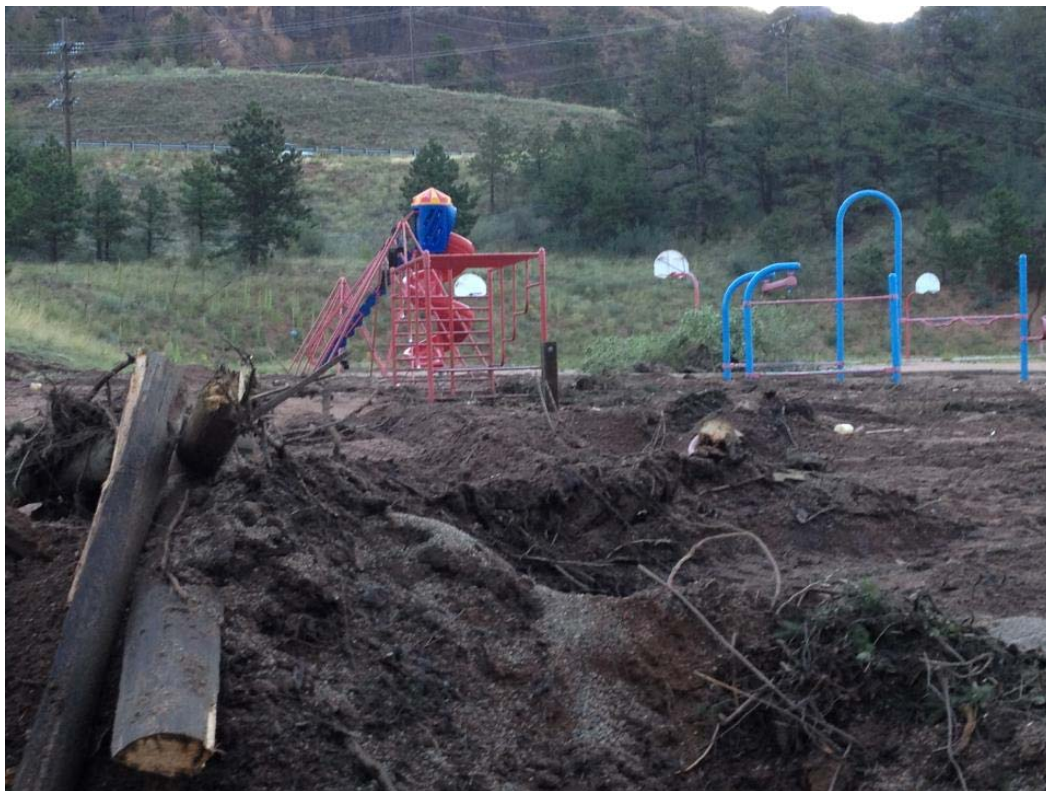
Figure 2. Ute Pass Elementary is threatened by flooding and debris from the Waldo Canyon burn area.
