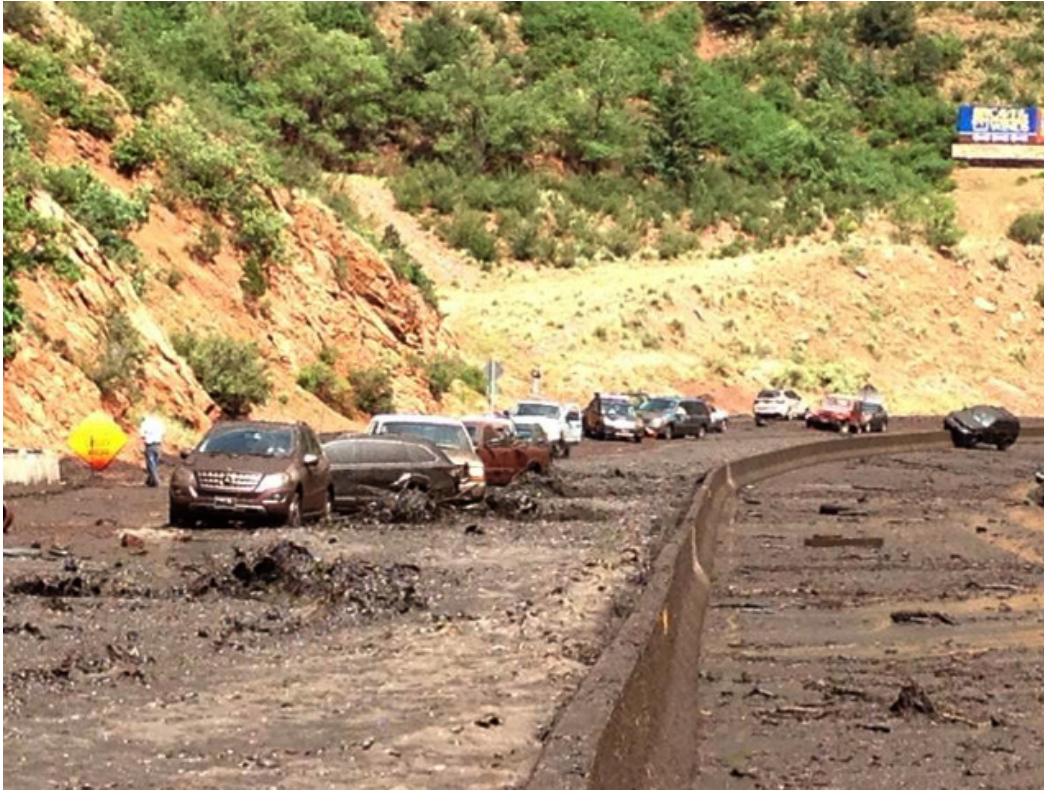
Figure 3. A flash flood off the Waldo Canyon burn area cripples Hwy 24 and takes the life of a motorist.
