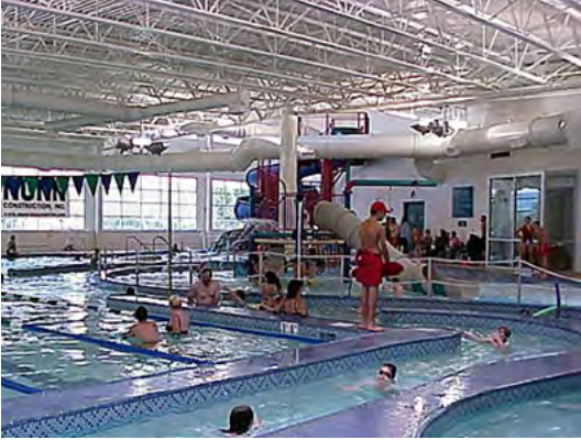
Memorial Park Recreation Center aquatics area. Source: City of Colorado Springs
