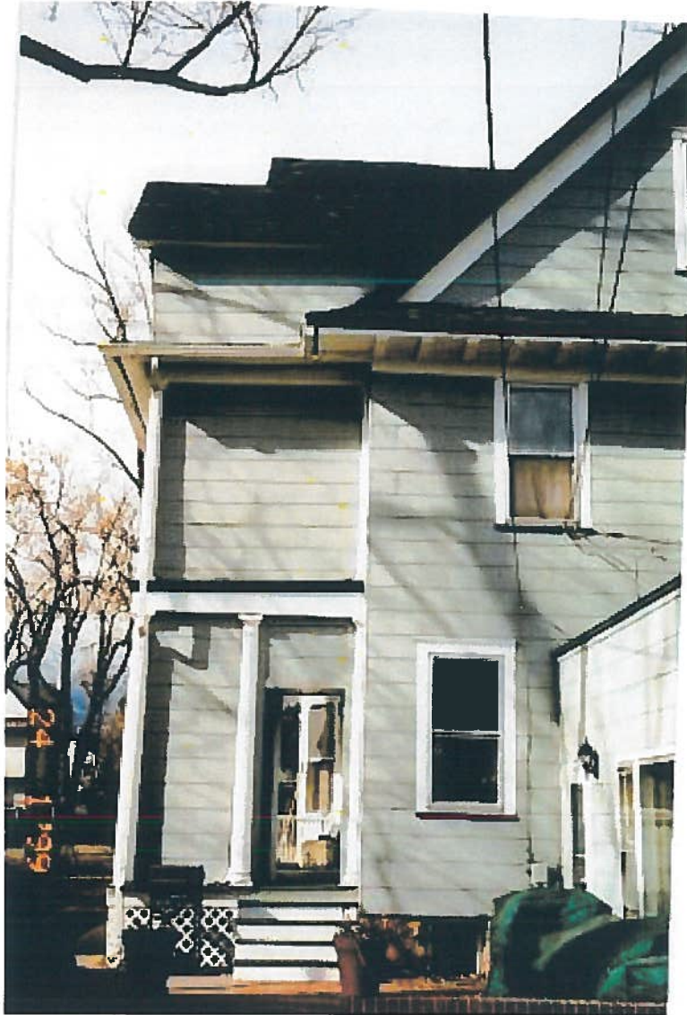
View of the rear of the porch and old window in what is now the master bathroom. This window was increased in size as part of the renovation.
