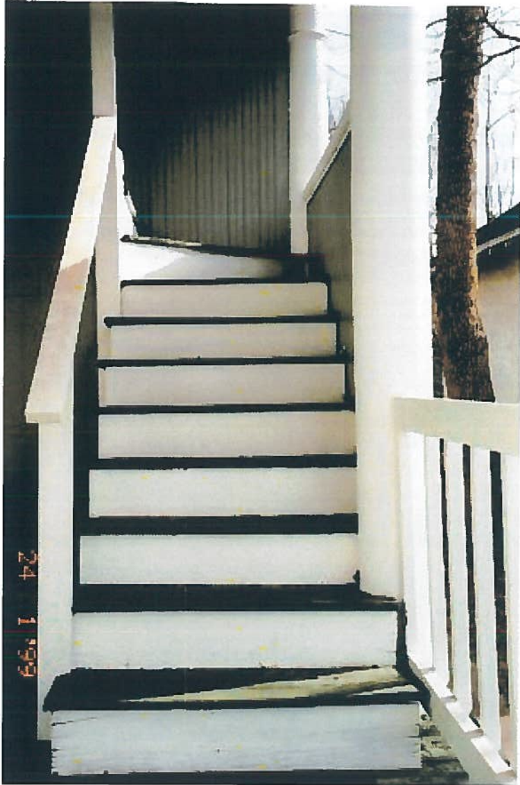
Stairs leading up to the former 2 nd and 3 rd floor apartments
