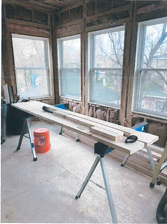
Current view from inside sunroom
