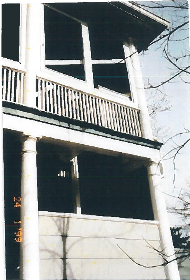
View of southern wall of porch
