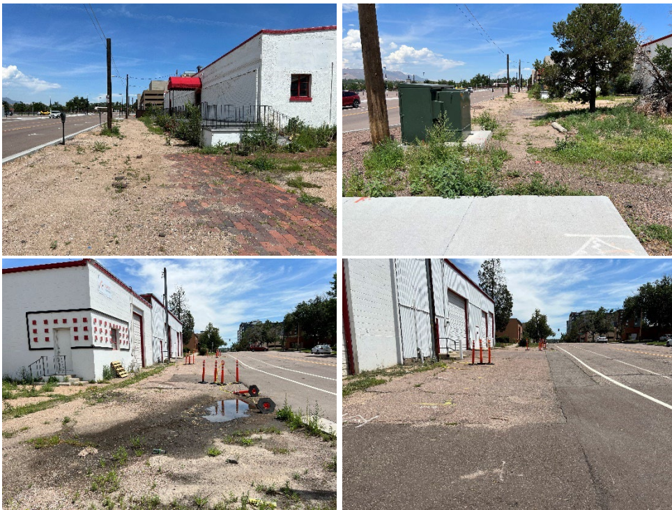
Figure 3. Poor Provision of Street Improvements for Pedestrians
