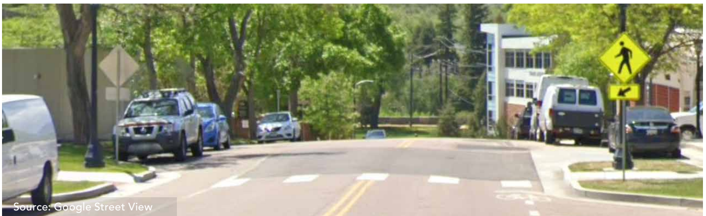
Mid-block crossing with elements that make it more visible and curb extensions to reduce crossing distance on Cache la Poudre Street.
