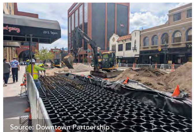
Soil cell installation along Tejon Street
