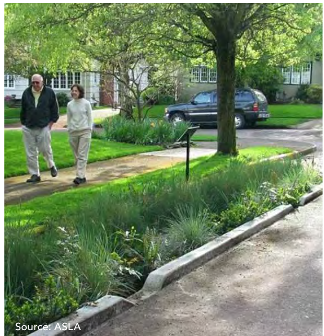
Low Impact Development (LID) infrastructure adds beauty, stormwater mitigation, and water quality improvements to neighborhood streets as shown in Portland, Oregon.
