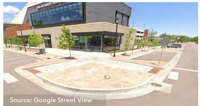
Curb extension reducing turning radius at Tejon and Dale streets.
