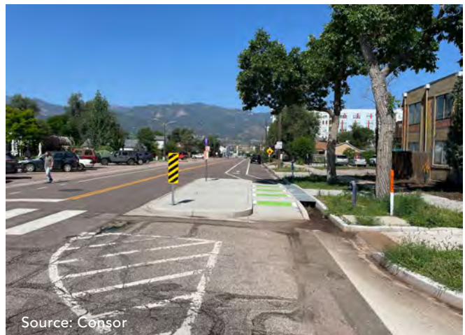
Bus bulb combined with bike lane on Rio Grande Street.
