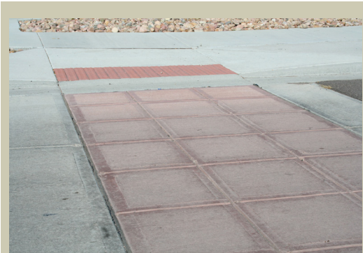
Figure 4.1-G. University Village Crosswalk
