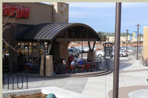
Figure 5.6-A. Example Photos of Building Entrances
