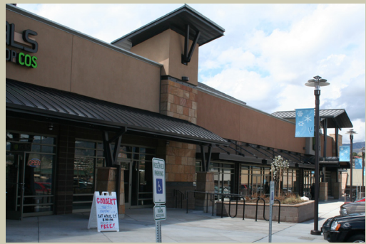
Figure 6.3-A. Example of Multi-Tenant Retail Facade
