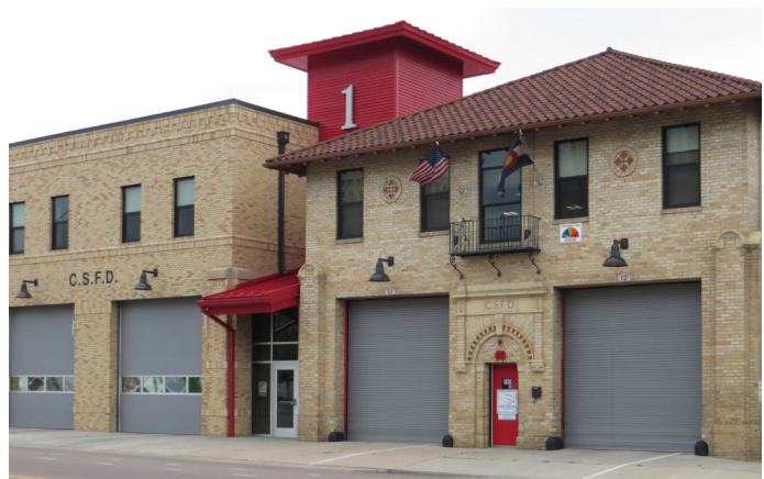
Figure 6: Fire Station No. 1, in service since 1925, was remodeled to create more space for equipment and brought up to code in 2016.
