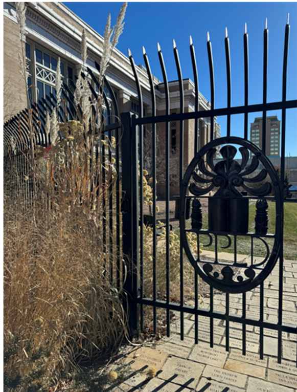
Existing fencing at Penrose Library
